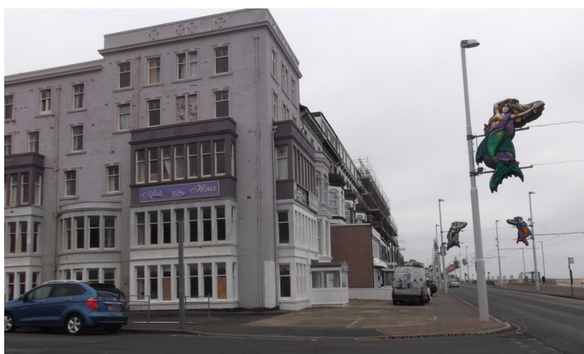
Figure 5: A dilapidated B&B in central Blackpool
